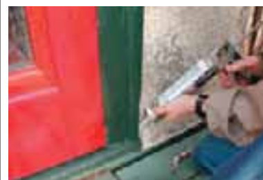
Caulk cracks and weatherstrip windows and doors to eliminate easy paths of entry. Check your foundation for cracks or spaces.
